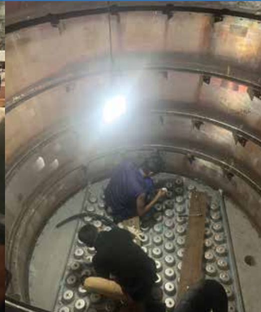
Installation and Testing Works of supplied internal parts of Medium Pressure Absorber (MPA) at Chittagong Urea Fertilizer Limited (CUFL)
