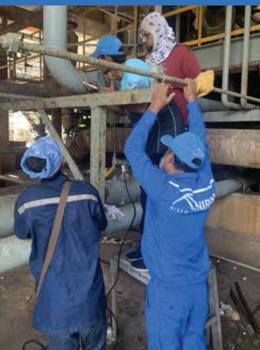
Installation of Discharge Valve of Boiler Feed Water Pump at Ammonia Plant and works of Block Fitting of Ammonia Delivery Line at Urea Plant of Chittagong Urea Fertilizer Limited (CUFL)
