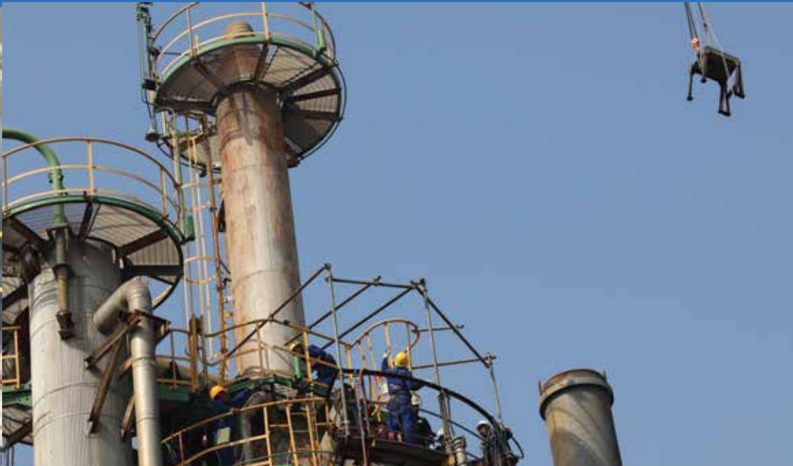
Ammonia Synthesis Converter Catalyst Unloading, Loading, Inspection, Basket Maintenance and Reduction of Ammonia Converter Project in Chittagong Urea Fertilizer Limited (CUFL)
